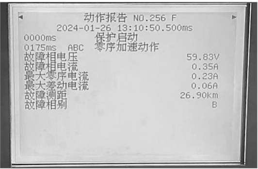
图2 故障瞬间动作报告 Fig. 2 Operation report at instant of fault
